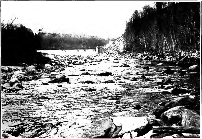
B. DAM OF GREENFIELD ELECTRIC LIGHT & POWER CO. ON DEERFIELD RIVER AT GARDNERS FALLS, BELOW SHELBURNE FALLS, MASS., NOVEMBER 27, 1911.
